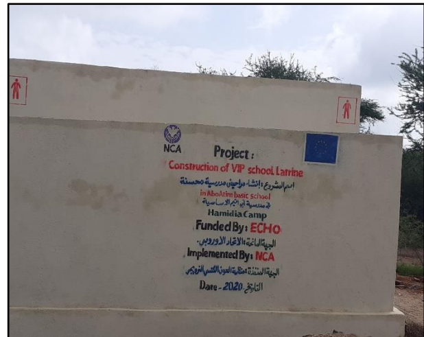
Figure 14: A constructed VIP latrine at the school by NCA in one of the camps
