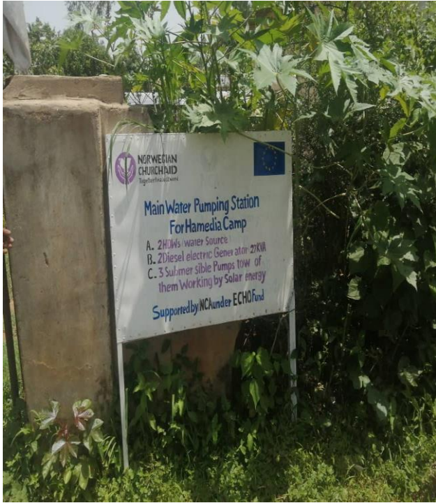
Figure 32: Main water pumping station
