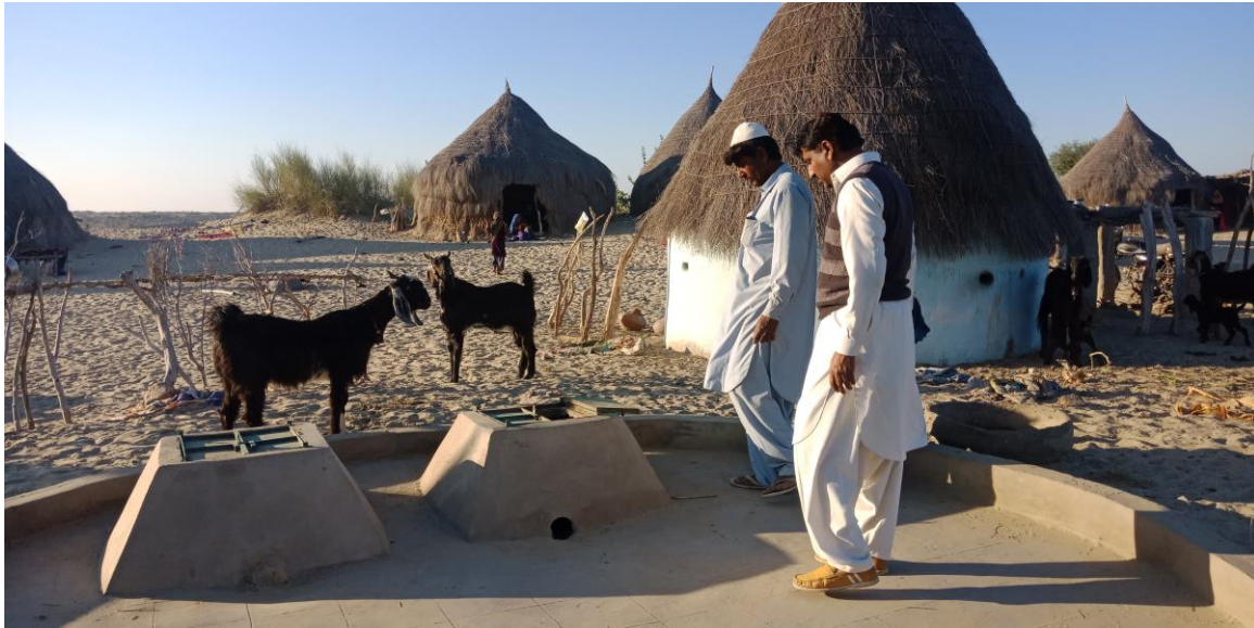
Picture 11: Rainwater Harvesting Storage
