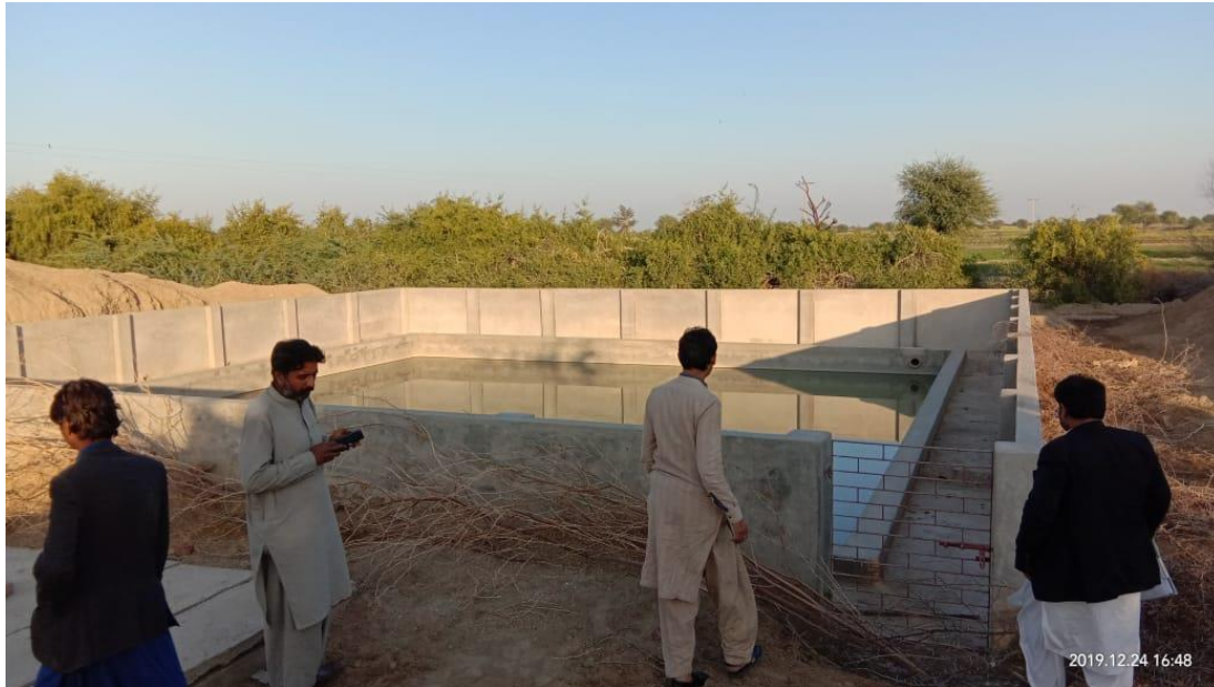
Picture 14: Water Storage Pond Constructed as part of the Programme
