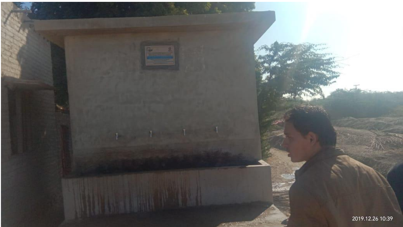
Picture 17: Water Tank Constructed as Part of Solarisation Initiative
