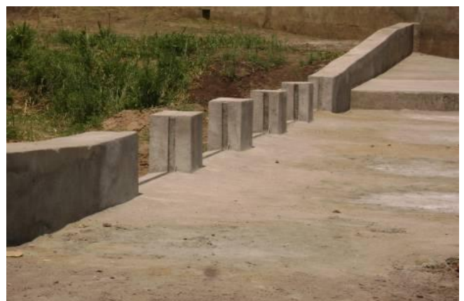
Figure 1 : Kwisa weir before and after rehabilitation
