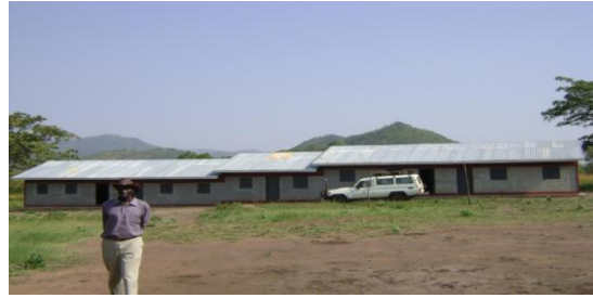
Photo 13 a school toilet that is disused
