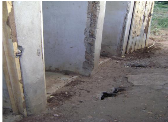
Photo 14 an incomplete toilet in one of the schools
