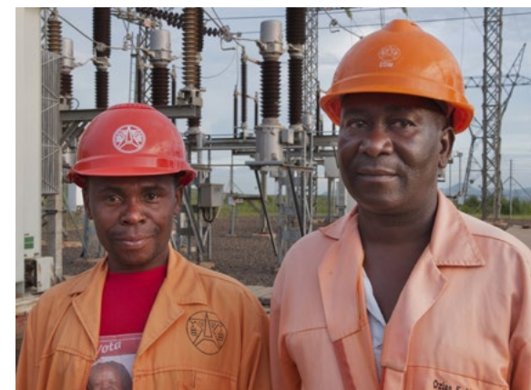
Lucas Lesta (TV) and Ozias Molane work at Lichinga Substation in Mozambique. PHOTO: Ken Opprann
