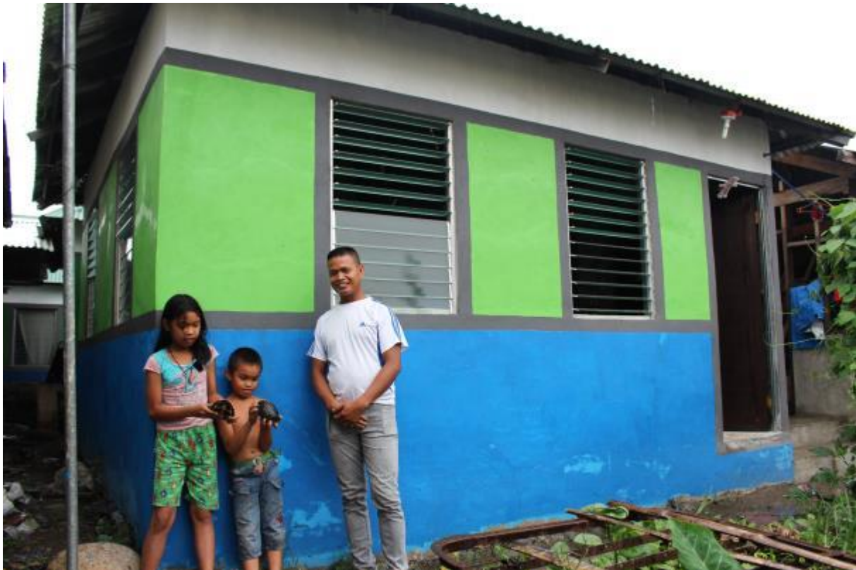
Figure 3: Onsite construction addressed some of the land access issues with these core houses built by LWR partner Habitat for Humanity. District 9, Bureau Barangay, Ormoc, Samar.
