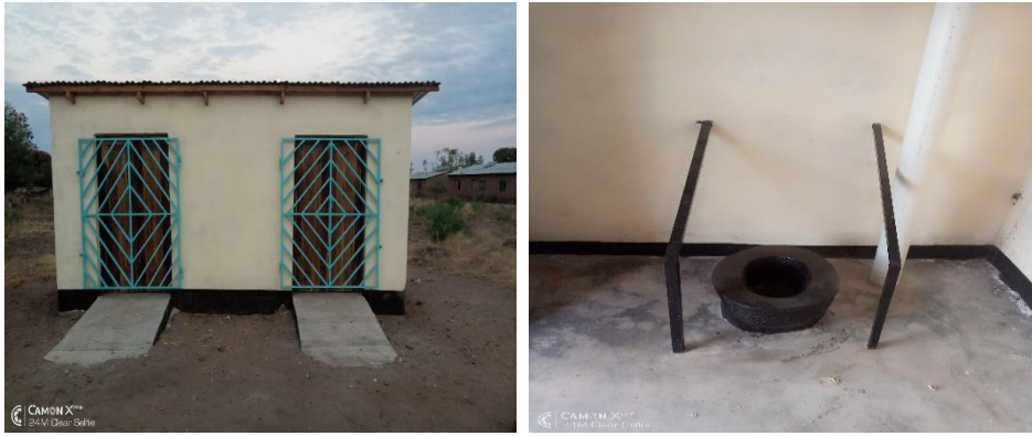
Above: Demonstration toilets constructed by the Safe Schools project for children with physical disabilities. Photo taken at Chiwondo Primary School in Karonga District.
