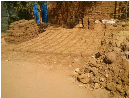
Photo 15 Local mud blocks used to rehabilitate or construct the learning shelters
