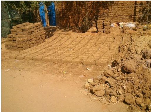
Photo 5 Local mud blocks used to rehabilitate or construct the learning shelters
