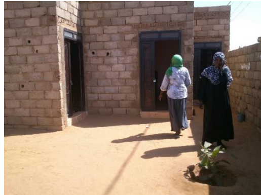
Photo 12 Three other rooms at the VTC
