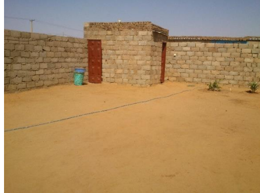
Photo 8 the two toilets constructed in a VTC
