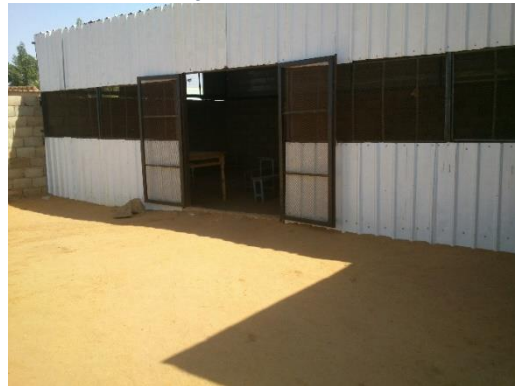
Photo 10 One of the rooms in VTC
