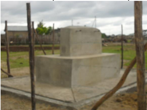
Photo 1. 5 Completed water collection point
