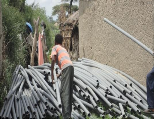
Photo 1. 1 the procured PVC pipes
