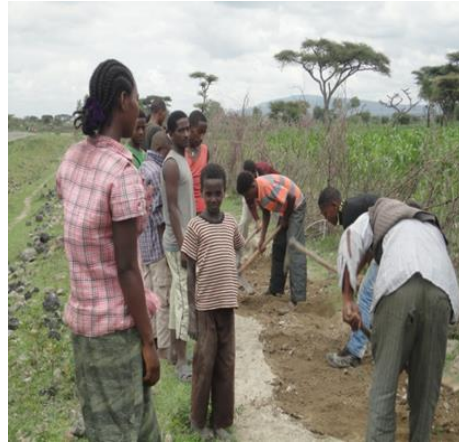
Photo 1. 4 Community members assisting in the laying of the pipes
