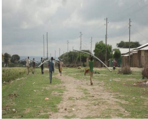
Photo 1. 2 community members helping in the laying of the pipes
