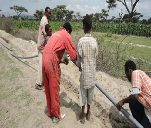
Photo 1. 3 The laying of the PVC pipes
