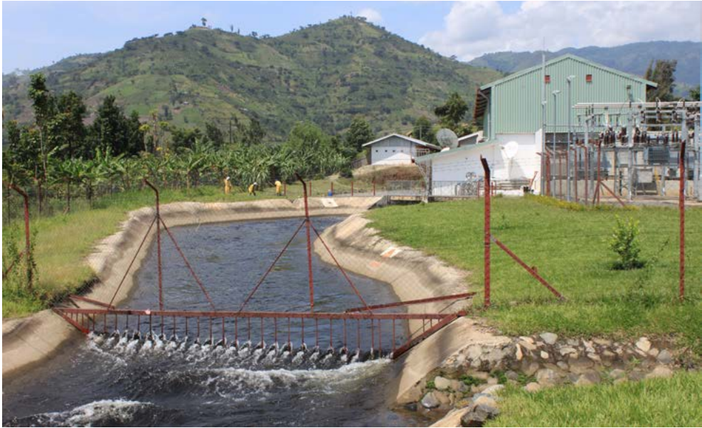
Bugoye power house. PHOTO: MORTEN SVELLE
