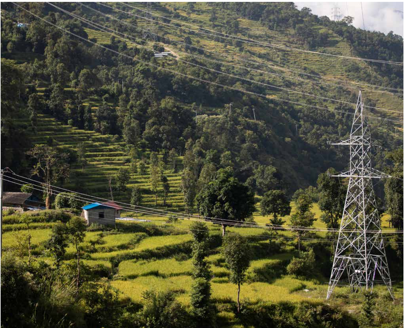
Power lines across rice fields in Butwal. Photo: Espen Røst
