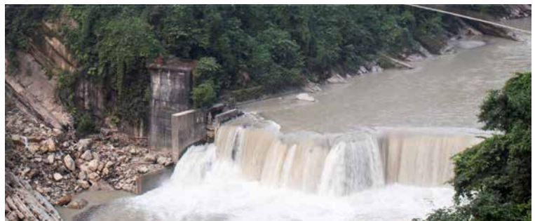
Now and then: Above, Tinau hydroelectric plant at the start of operation in 1978. Below, the Tinau dam in full operation today. Note the difference in water flow due to seasonal variation. Photo: HimalPartner and Espen Røst
