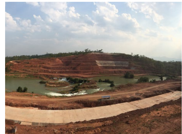
Dam site, Upper Keng Tawng Hydropower project PHOTO: FRIDA MARTINSSON (MULTICONSULT)
