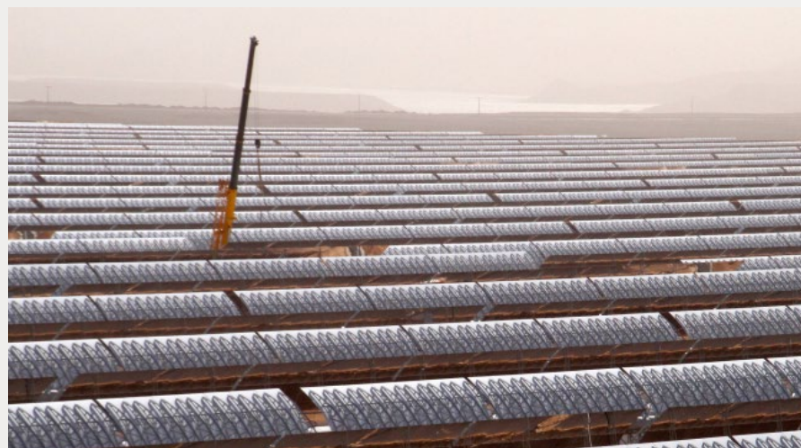
The first 160 MW of Noor-Ouarzazate Concentrated Solar Power complex. PHOTO: WORLD BANK
