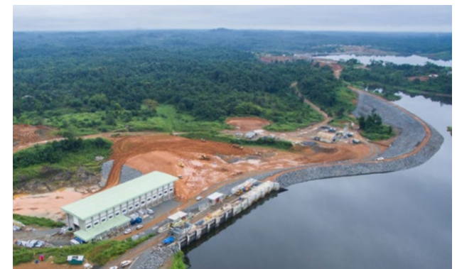
Mt. Coffee Hydro Power Plant in Liberia, Powerhouse. PHOTO: DAWNUS INTERNATIONAL
