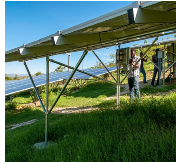
Installation of solar PV panels in Haiti PHOTO: UNEP
