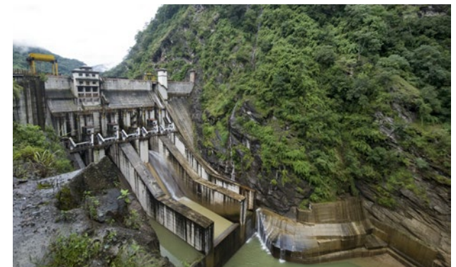
Bhutan Tala Hydropowerplant dam. PHOTO: KEN OPPRANN
