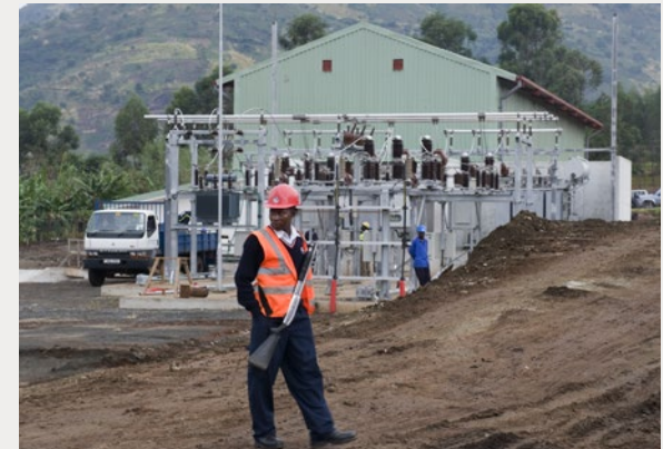
Bugoye power house PHOTO: KEN OPPRANN
