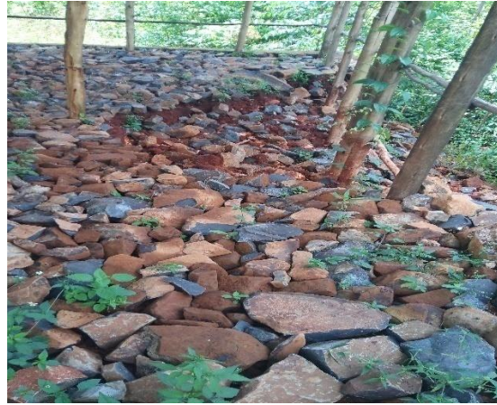
Photo 1: Assosa dairy farm damaged by flood
