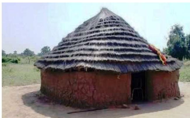
Plate 14 – Mayom PHCU (current structure)
