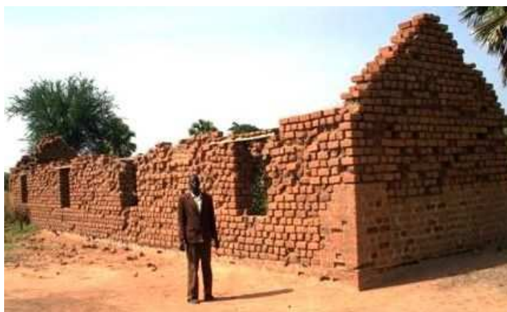
Plate 22 – Mayom PHCU (uncompleted current structure)
