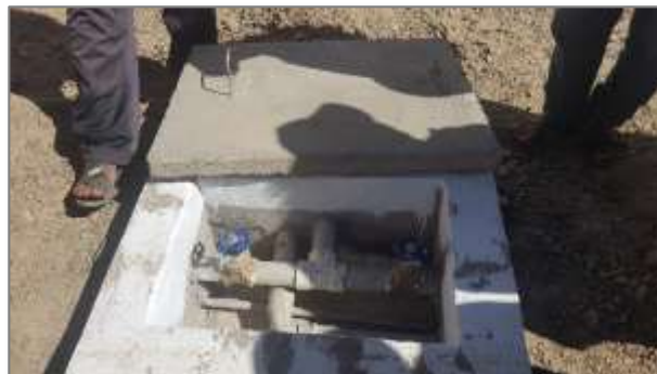
Image N° 8: Valves Chamber – Water System of the Community Collpani from the Municipality of Luribay (*)
