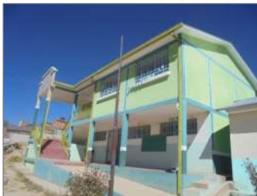
Image N° 2: Built Classrooms in the E.U. Republic of Venezuela from the Municipality of Luribay
