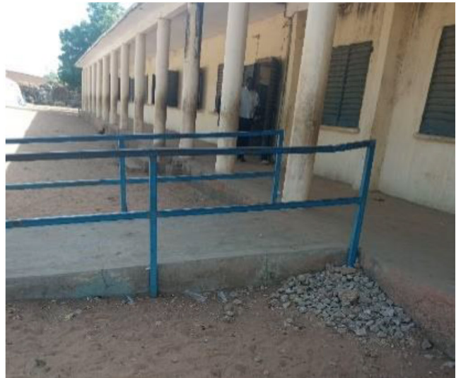
Access ramps to the Maradi Centre Primary School
