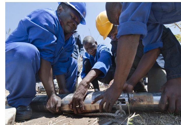
Water pipeline being repaired. PHOTO: KEN OPPRANN
