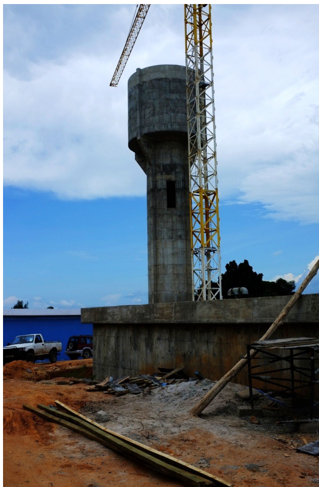
Picture 2 – ZAWA's new water storage project in Chake Chake
