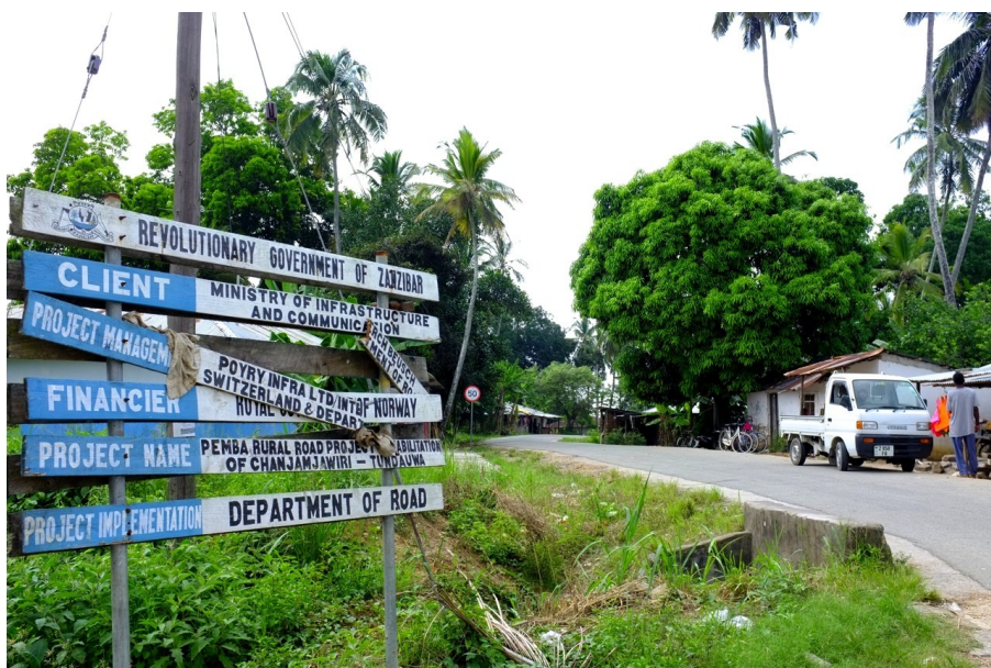
Picture 1 – The Chanjamjawiri-Tundauwa road
