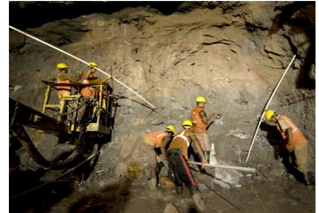
Tunnel drilling and blasting. PHOTO: KEN OPPRANN
