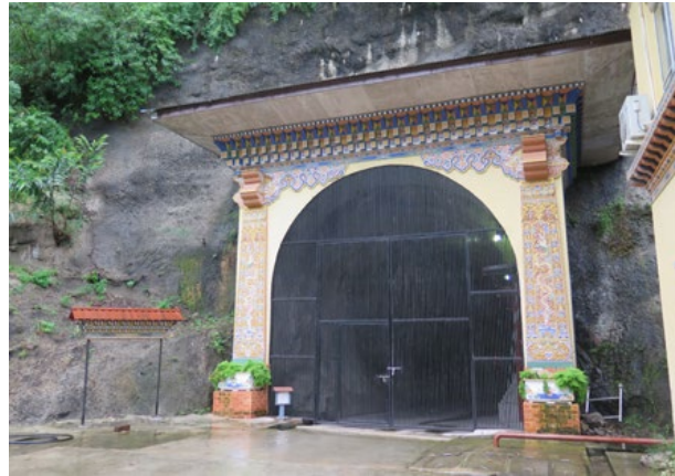
Dagachhu hydropower plant. PHOTOS: HARALD BIRKELAND
