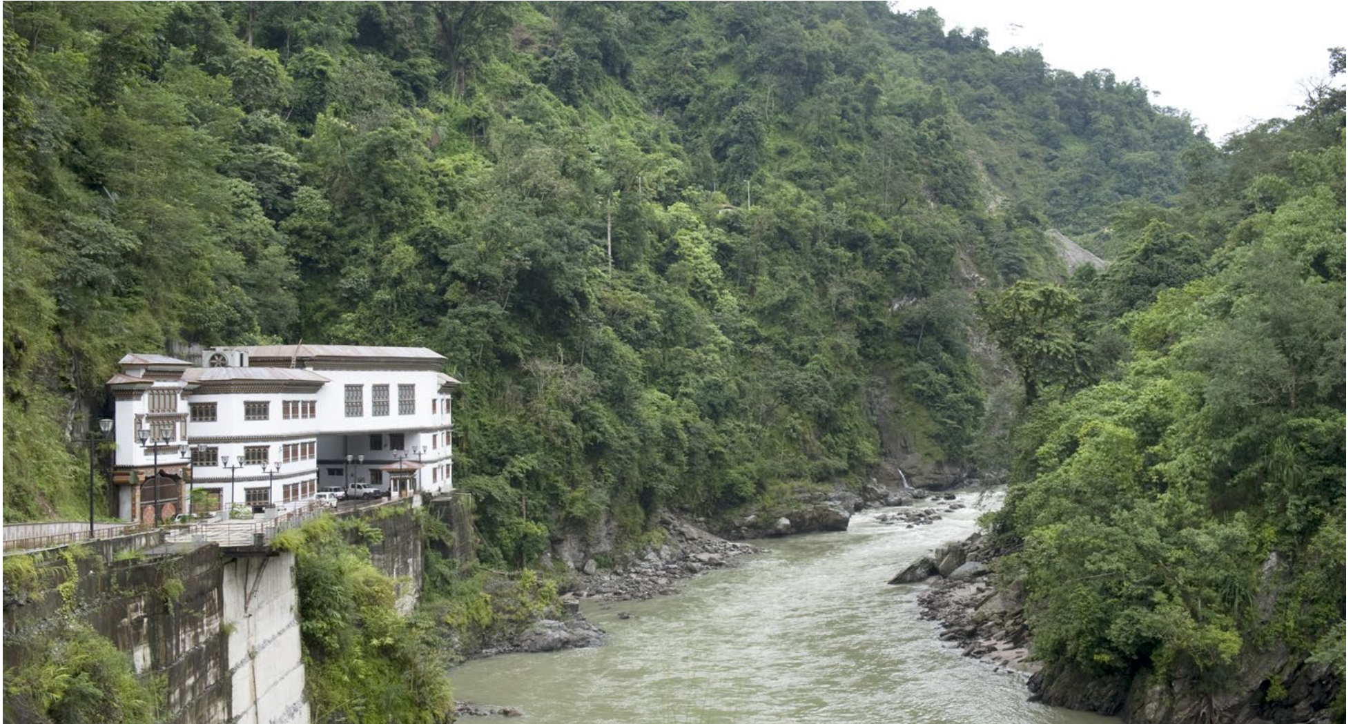
Tala hydropower plant. PHOTO: KEN OPPRANN
