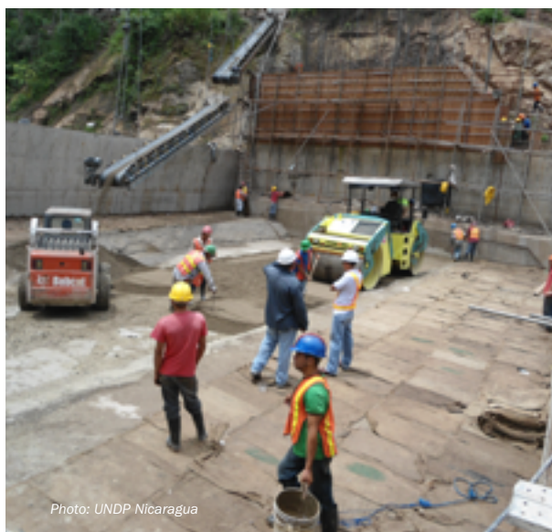
Construction of a small hydroelectric station in Wiwili, Nicaragua.
