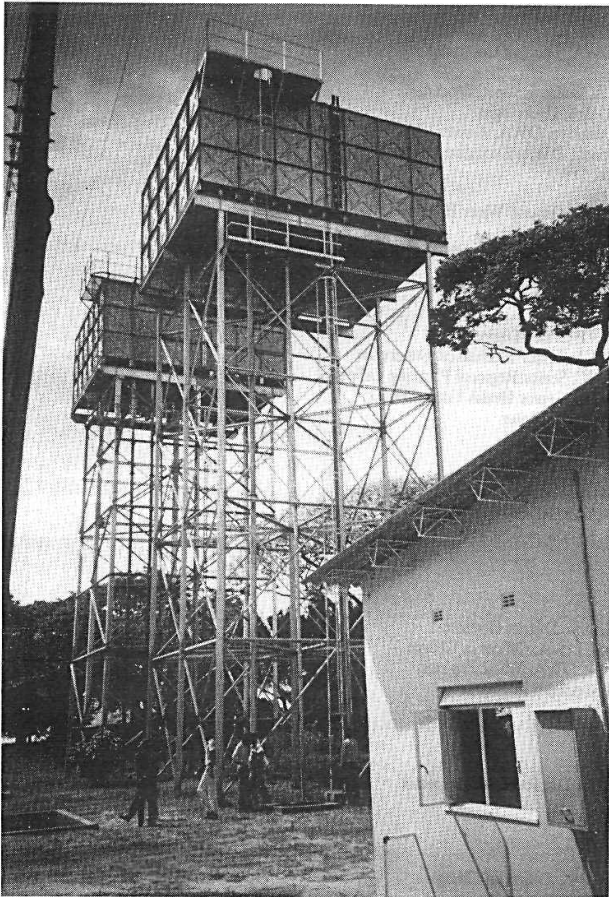
Details from the township water supply in Kalabo
