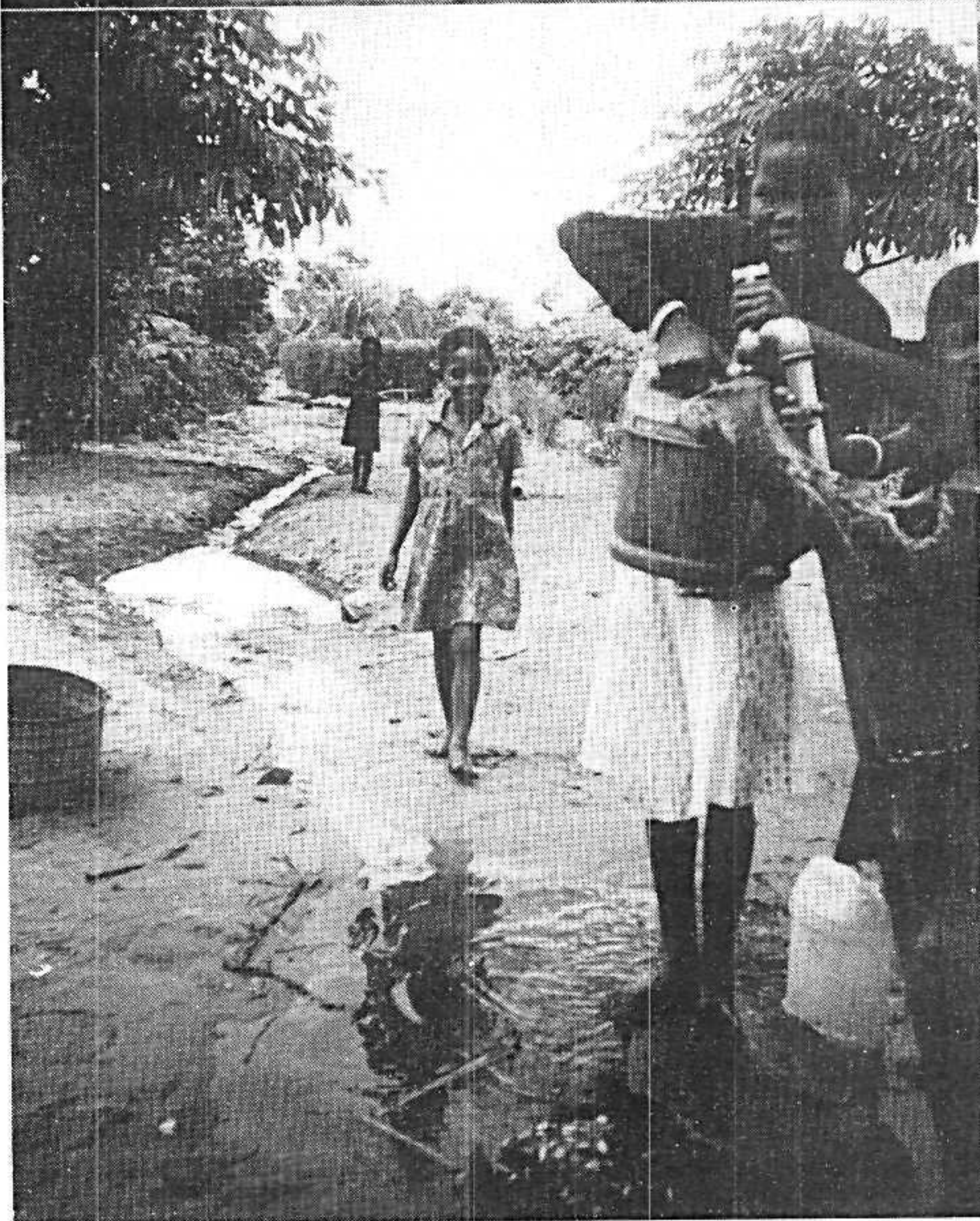
Details from communal standposts, Mongu township water supply scheme. The pipes are very vulnerable since there are no headworks, and the surroundings are unhygienic since there are no run-offs or soak-aways.
