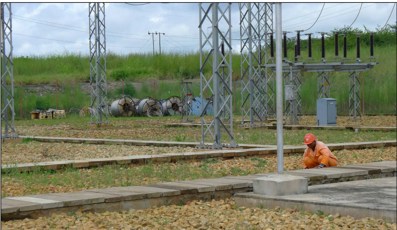
Picture 3. Vegetation clearing at Metoro substation.
