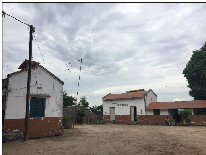
Picture 6. Health Clinic in Bilibiza previously supplied with solar PV
