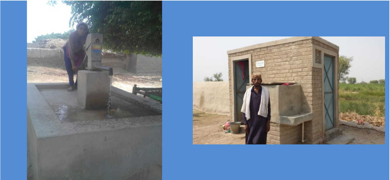
Project Supported Hand Pump and Latrine Set
