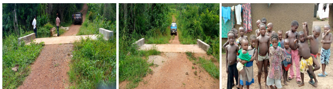
CELAD Infrastructural project (Two bridges constructed) at Gondama in Moyamba District
