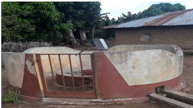
Water well project at Gandonhun –Bo District
