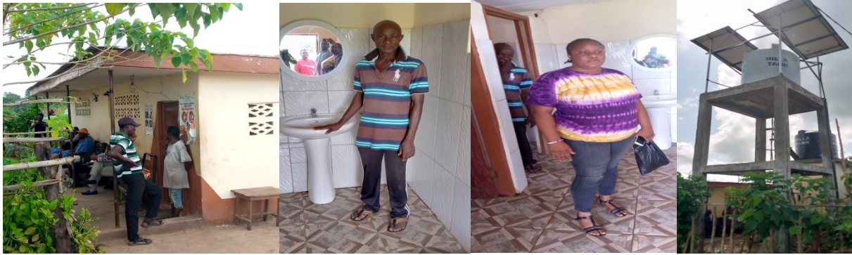
CELAD Health project (Community toilet constructed at Tiama in Moyamba District)
