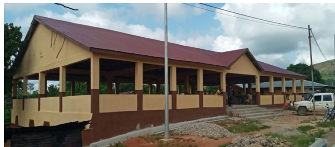
Completed Market at Panguma in Kenema District
