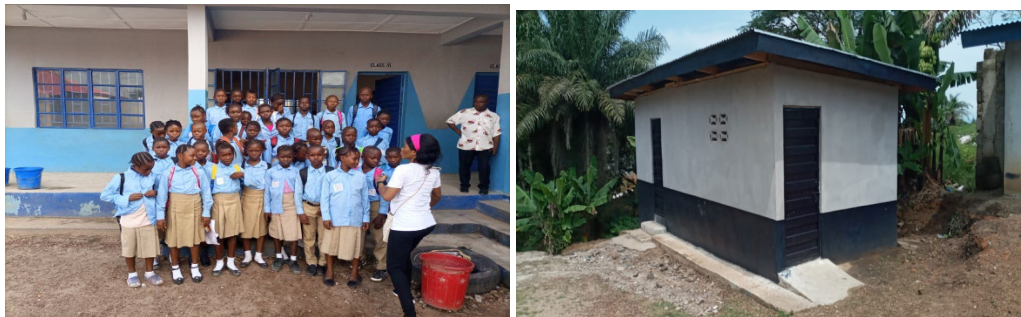
Completed school building in Magburaka - Tonkolili District
