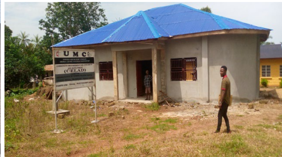
Construction of a training center in Yonibana
