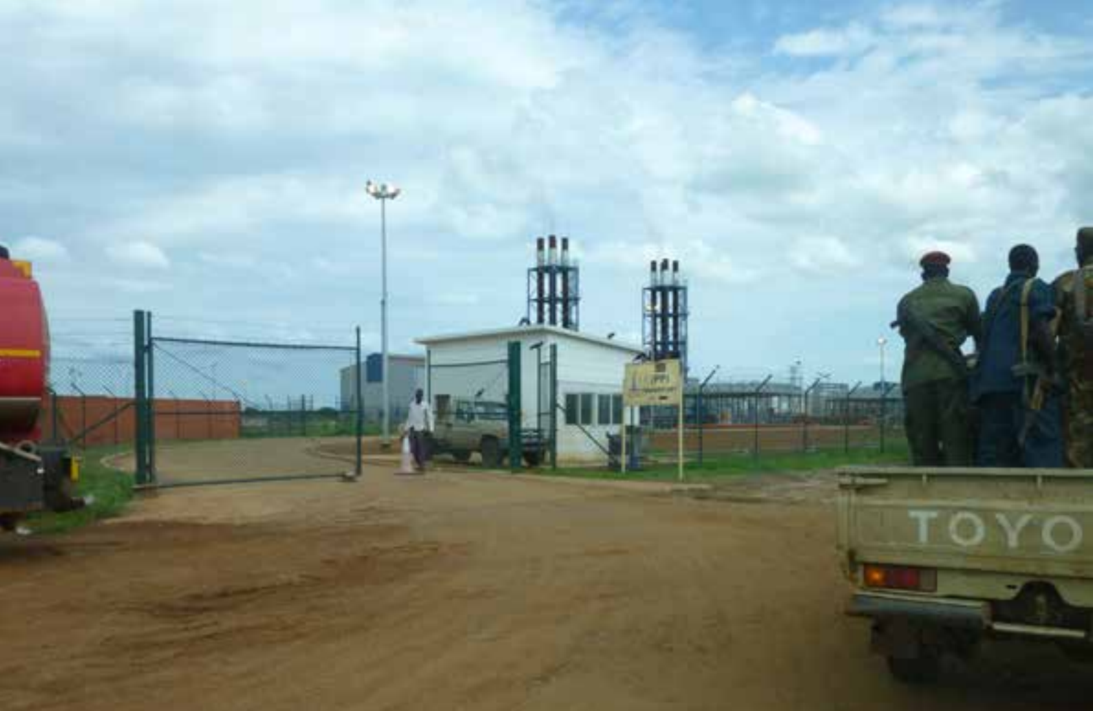
Oil power plant providing electricity to the oil installations in the Upper Nile, South Sudan. Photo: Stein Paul Rosenberg
