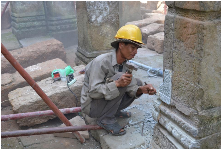
Worker at the Taprom Temple Restoration Site, Siem Reap
