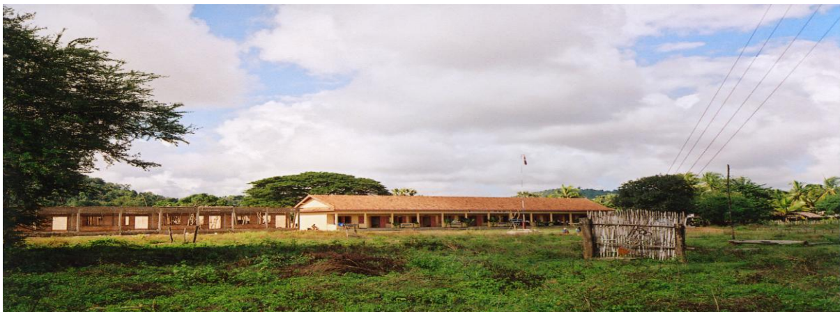
Lower Secondary School under construction at Kompong Srolau, Chheb District alongside the Primary School
