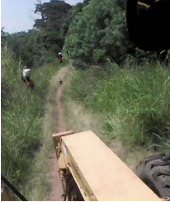
The road before construction. PHOTO: CARITAS NEBBI
