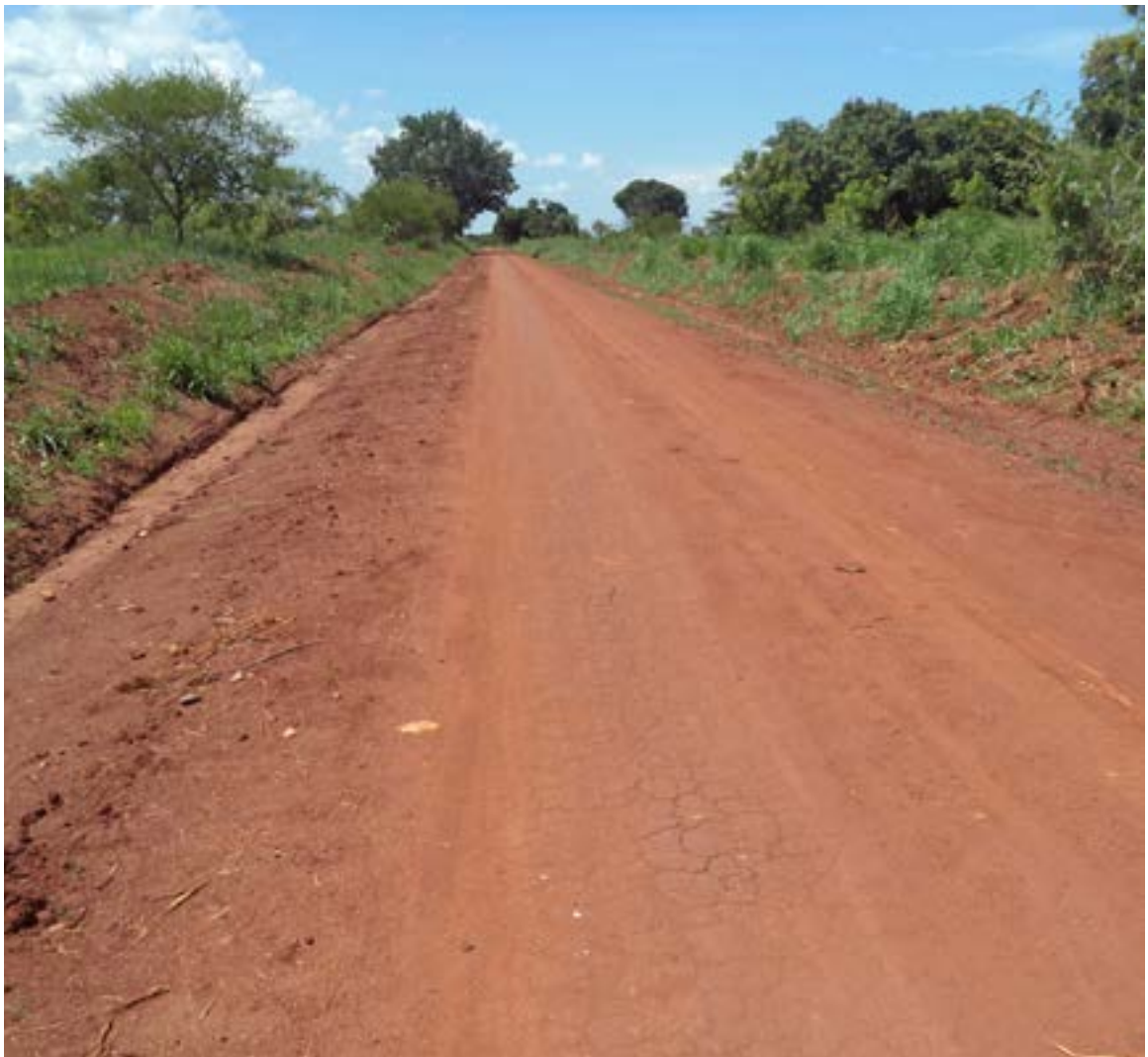
The access road after construction. PHOTO: CARITAS NEBBI
