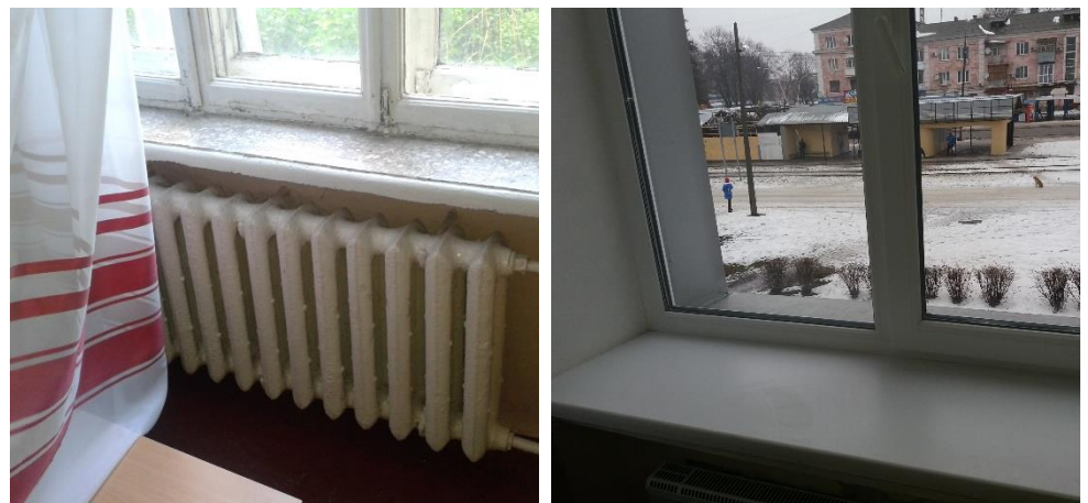
Figure 3. Replacement of windows and radiators
