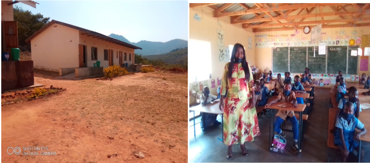
Left Photo: Completed classroom block at Saungweme Primary School Right Photo: grade one pupils captured enjoying learning in the new classroom block
