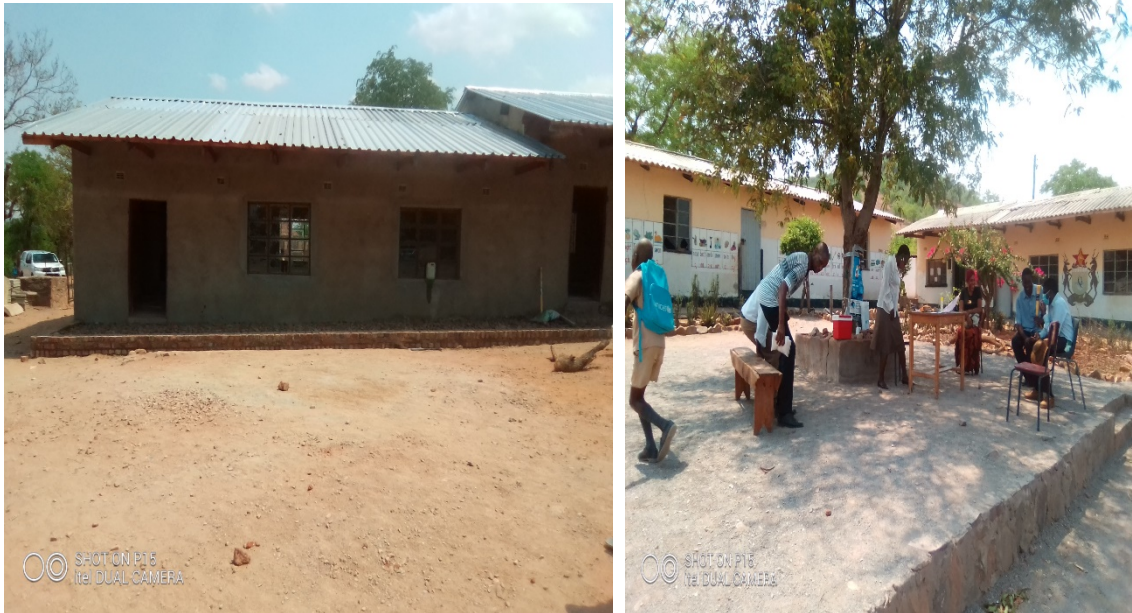
Left Photo: Classroom block under construction at Nenhowe Primary School
