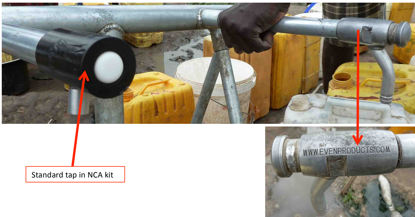
Figure 2.1: Showing the black & white standard tap being standard on the water supply distribution tap stand in the NCA kit. This easily breaks, and the module should be mounted with more sturdy metal taps, e.g. from Even Products in UK (photo from Gumuruk, South Sudan).
