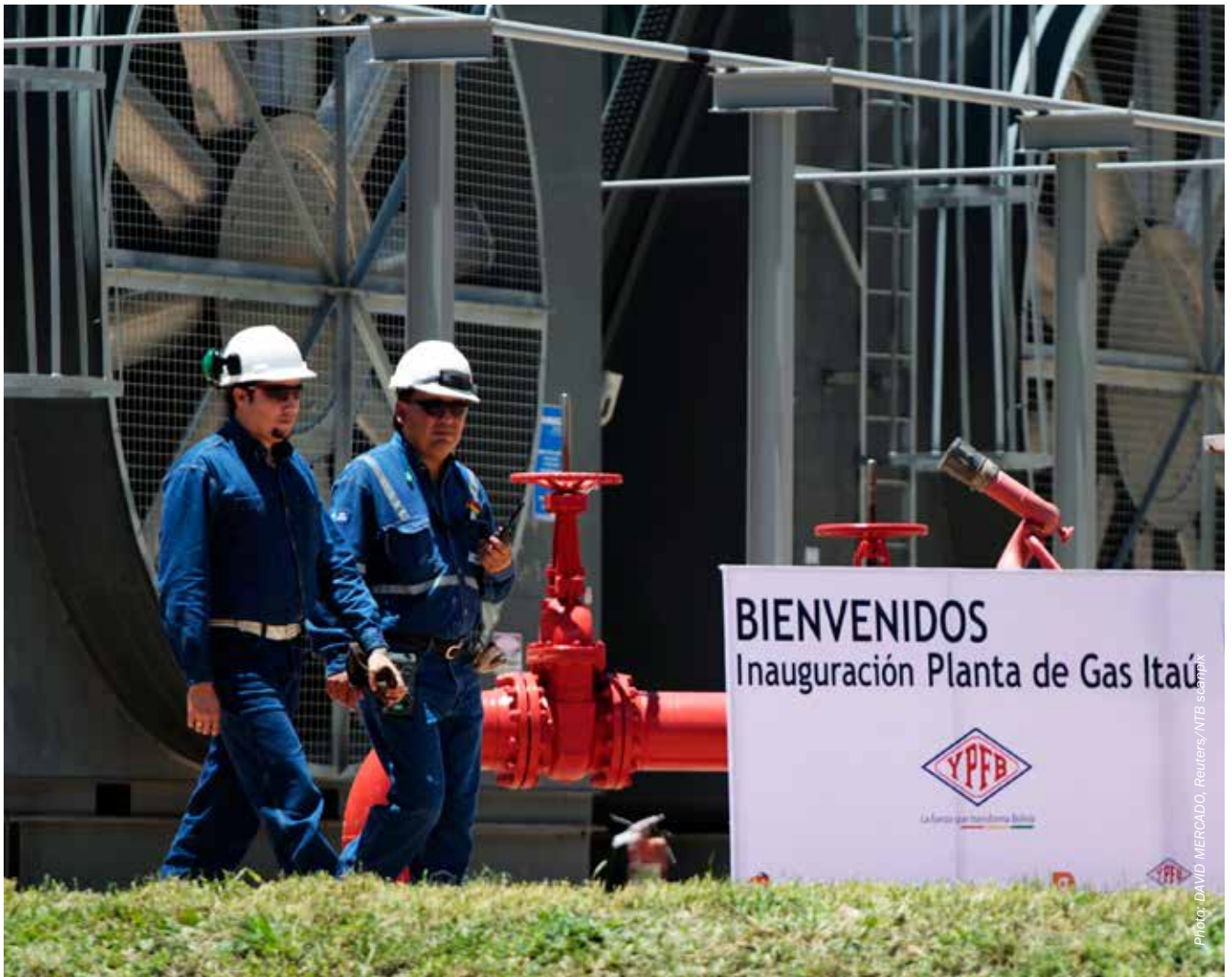
Oil workers at Itau Natural Gas Processing Plant in Carapari, Tarija province, around 750 km south-west of La Paz.
