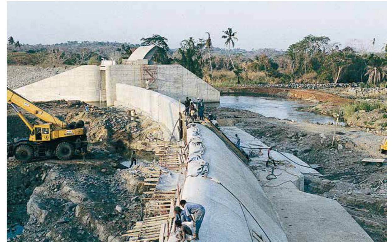
Pangani Dam under construction. Photo: Norplan/Multiconsult (1994)
