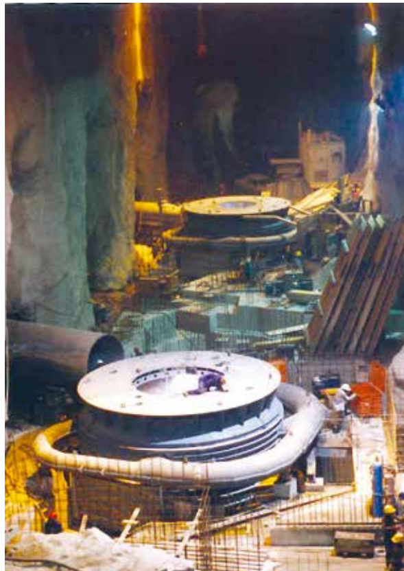
Pelton turbines from Kværner being mounted at Kihansi. Photo: Even Sund (1998)
