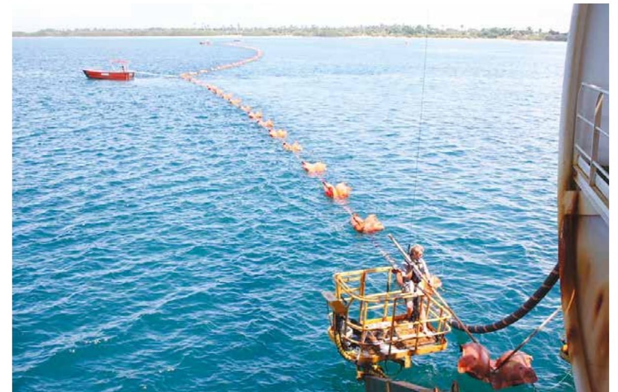
The sub-sea cable brought ashore on Pemba. Sea levels vary significantly at high and low tide, meaning that the work had to be meticulously planned and executed. Photo: John Alvsvåg (2009)
