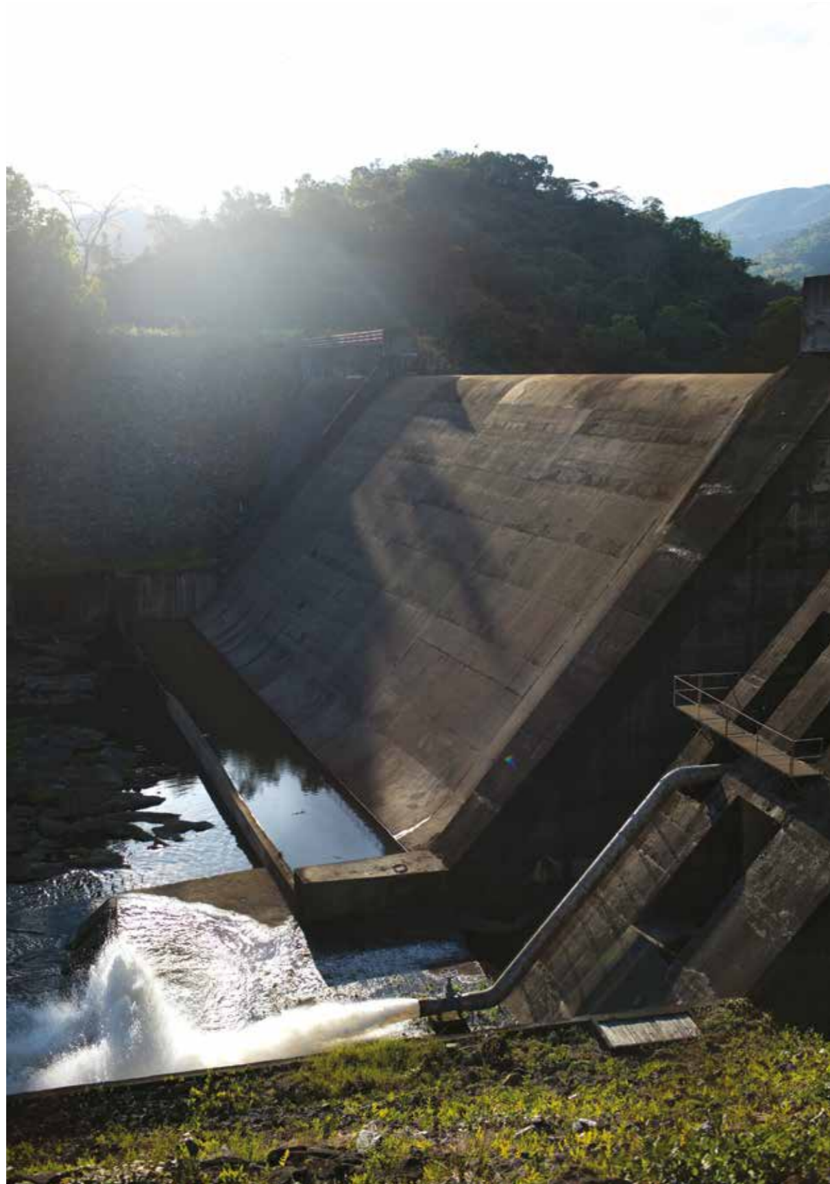
Kihansi Hydropower Plant. Photo: Espen Røst (2019)
