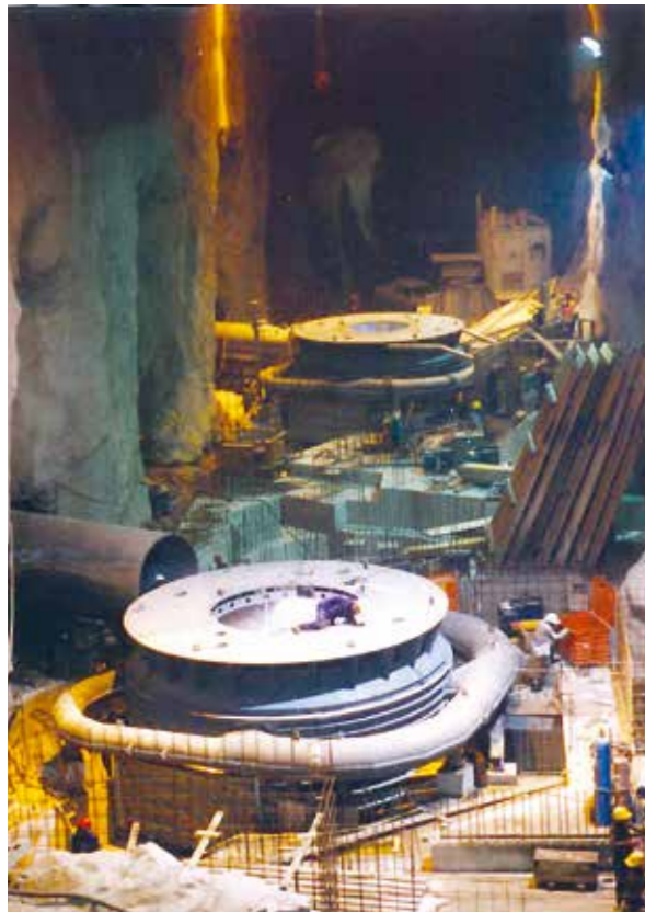
Pelton turbines from Kvaerner being mounted at Kihansi. Picha: Even Sund (1998)
