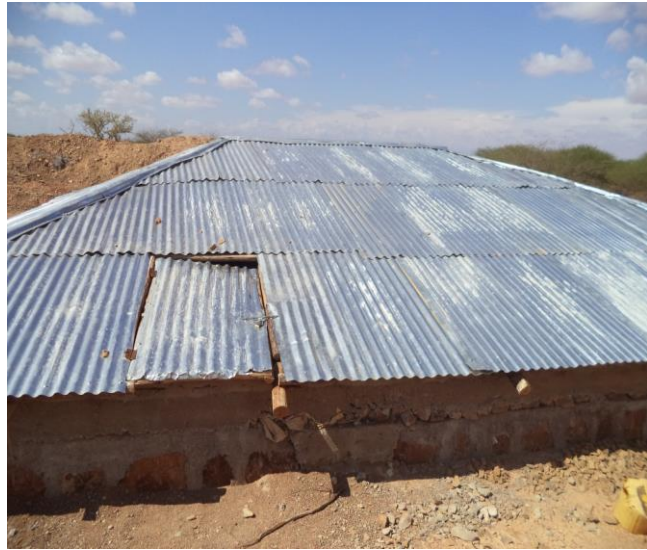
Rehabilitation and roofing at Adajigo community
