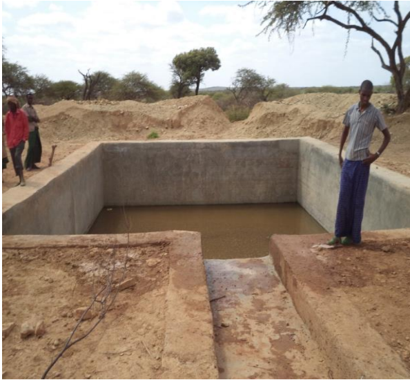
The new birka constructed in 2013 at Hasse gabey community
