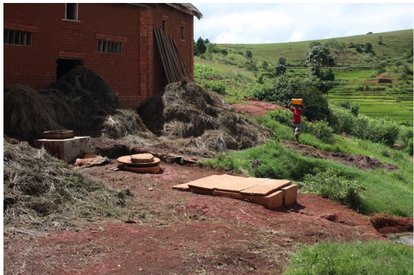
A biogas digester outside the barn.
