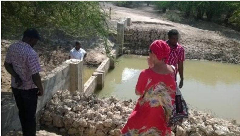
Figure 2: Site observation at inlet and outlet of Bangale Dam
