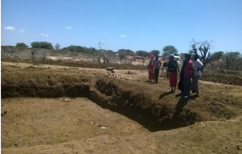
Figure 5: The paused Bisanhargeisa proposed water cistern excavation work
