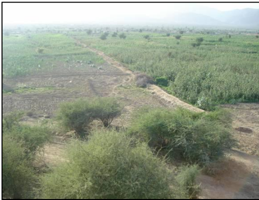
Fig. 12 Adi-Shuma Embankments & soil bunds
