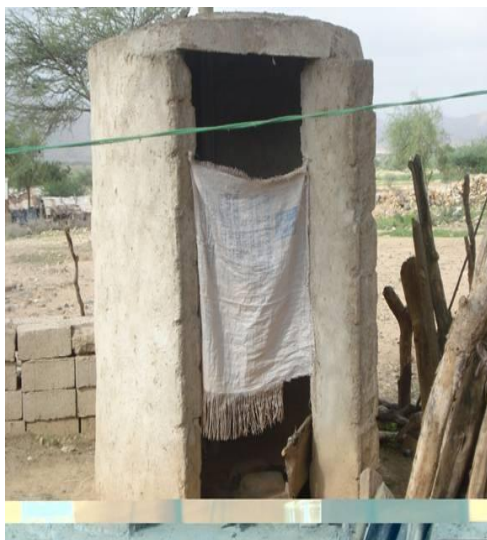
Fig.10 Pilot Latrine constructed by SDIDP
